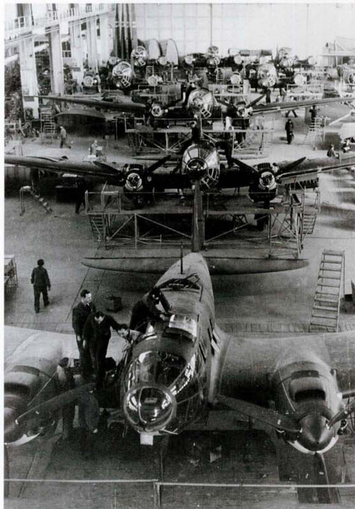
ABOVE AND ABOVE LEFT: A number of He 111 bombers and He 115 floatplanes under construction at the Heinkel factory at Rostock during 1939. Note that the aircraft already have their standard European camouflage and national insignia applied with their radio call signs (Stammkennzeichen) painted in white on the fuselage sides. The He 111 nearest the camera is W.Nr. 2921, NA+IT.
