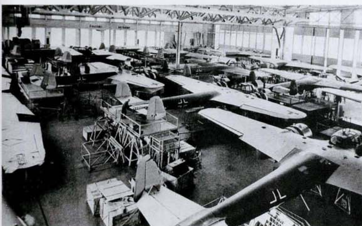
ABOVE: A batch of Do 17 Zs under construction. At this stage most of the basic camouflage and national insignia have already been applied. It only remained for the operational unit to which they were delivered to apply its own identity markings.
